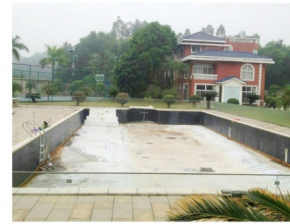
1. 基面平整 Surface smoothing
