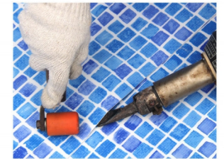
6. 池底铺设焊接 Floor laying and welding
