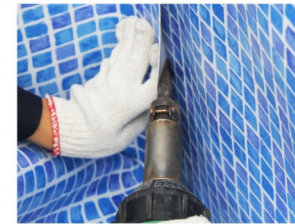
5. 池壁铺设焊接 Wall laying and welding
