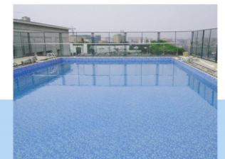
9. 试水验收 Acceptance inspection
