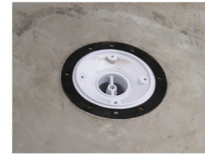
2. 泳池功能件预埋 Installation of embedded parts
